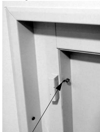
Figure 8: Secure to door frame
